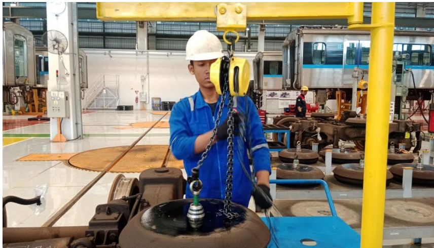
Gambar 10. Pemasangan alat crane trolley jig air spring
