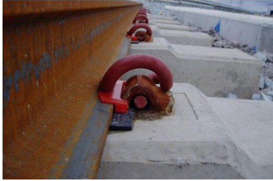
Sumber : Pandrol.com Gambar 2. Penambat Elastis E-Clip
