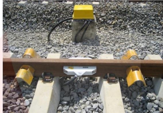
Gambar 2 Peralatan luar *axle counter double head*
