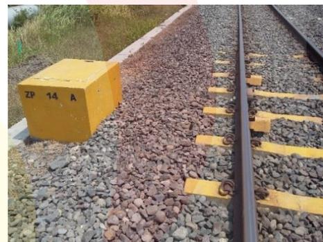
Gambar 3 Peralatan luar *axle counter single head*
