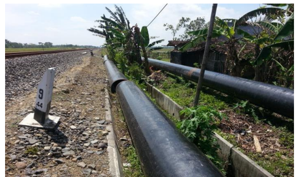
Figure 2. The Preparation of placement pipelines beneath railway tracks
