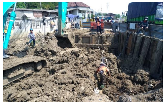
Figure 3. Excavation Process Of Placement Pipelines beneath Railway Tracks
